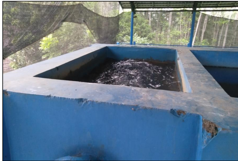
Gambar 4.27. Bak Intake Building
